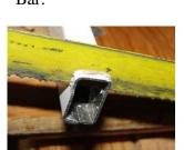
2. Cut the Brace bar with a hack saw. It is best to wrap the section of the Brace Bar you are cutting with clear tape to guard against accidentally scratching the paint with the hack saw. Test the fit of the brace bar between the patio screen frame rails. Re-cut if needed.
