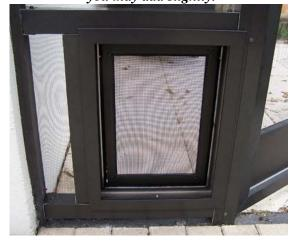
7. Once the pet door is installed you can fill any gaps or seal the edges with caulking if desired.
