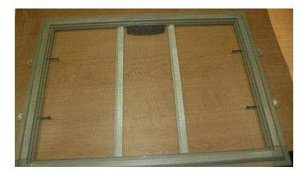
D) Starting at one corner using your fingers start the screen spline into the screen bar, then using the concave end of the screen roller tool slowly roll the screen spline into place.
